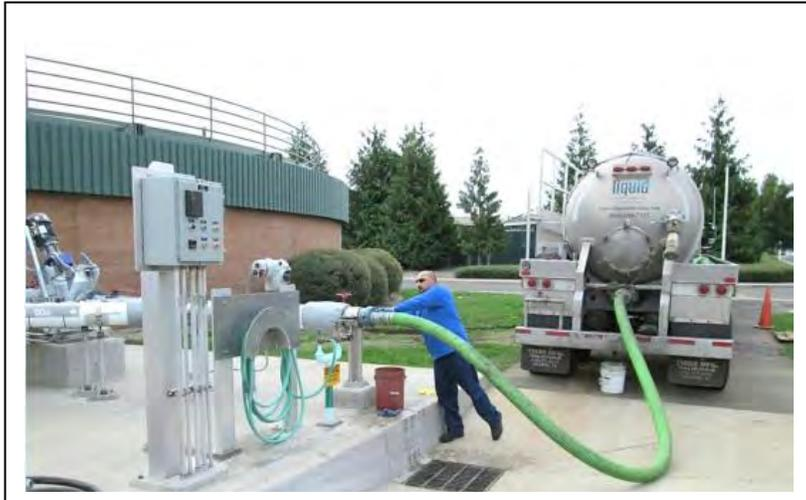
**FOG Receiving Station. The Gresham WWTP Doubled Biogas Production by Collecting about 12,000 gallons/day of Fats, Oils, and Grease (FOG)**
