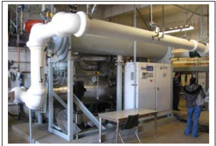
**280 kW binary Pratt & Whitney PureCycle ORC powerplant at OIT (Geo-Heat Center)**
